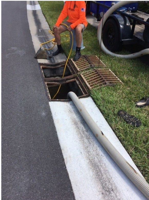
SWM - Drainage Structure
