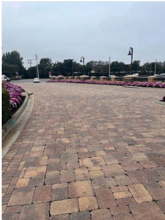
Entrance - Roadway & Lighting
